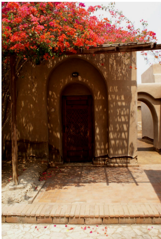
Figure 5 The unsuccessful preservation works undertaken to the buildings in the art centre [19].
